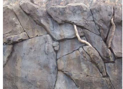
The project, located at the intersection of Oatfield Road and McNary Road in Gladstone, Oregon, required construction of three separate wall types: Soil nail, soldier pile, and cantilever with conventional footing. Each received the carved shotcrete treatment, providing a consistent, natural appearance.
